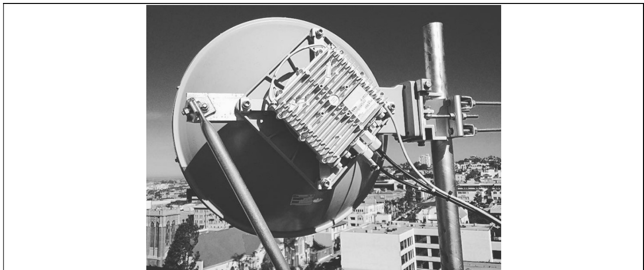
FIGURE 4a: 2FT Antenna installation (EH-ANT-2ft-B)
